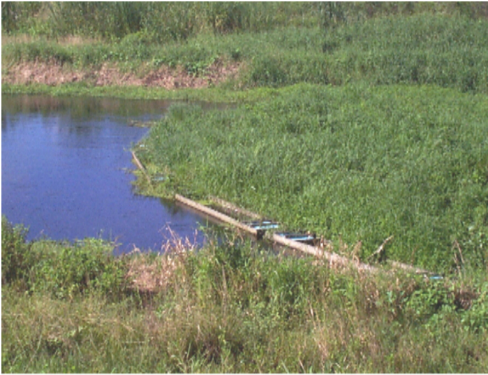
Figure 5. Hyacinth barrier installation.
