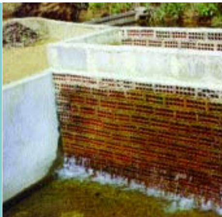
Figure 79 A simple gravel filter on a farm supply system helps to exclude predators (Brazil)
