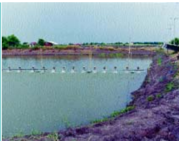
Figure 64 Long-shaft aerator in action (Thailand)
