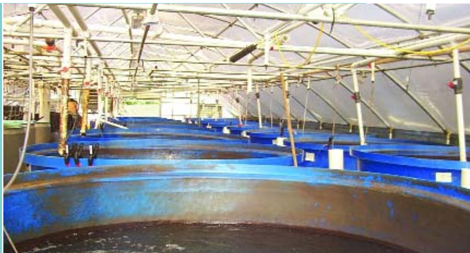
Figure 38 Overhead air and water distribution systems are used to supply these indoor nursery tanks (USA)
