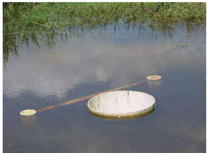
Figure 7.12. During the production season, ponds should drain from the surface, not the bottom, to minimize disturbance of surrounding drainages and watersheds.
