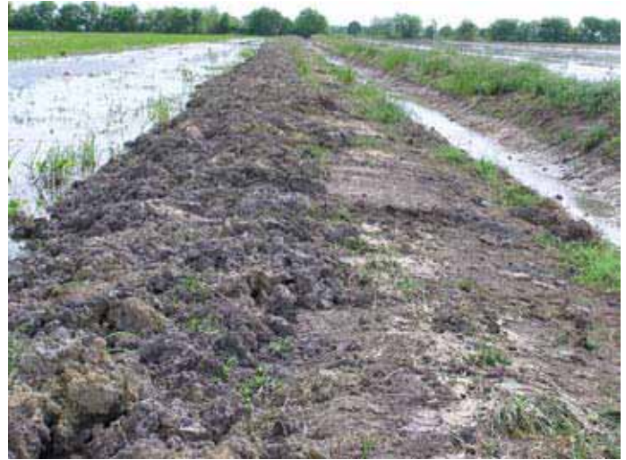
Figure 7.17. Drainages that are managed to capture solids as they leave production ponds can often provide a ready source of soil for levee maintenance.
