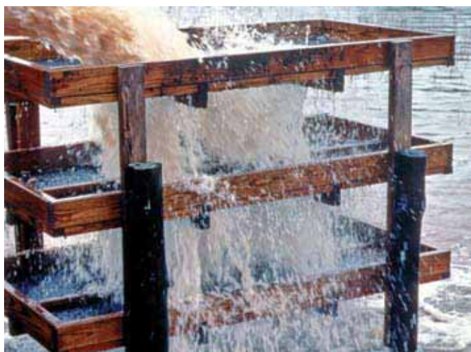
Figure 7.1. Well water, while usually free from contaminants, must be vigorously aerated prior to use.
