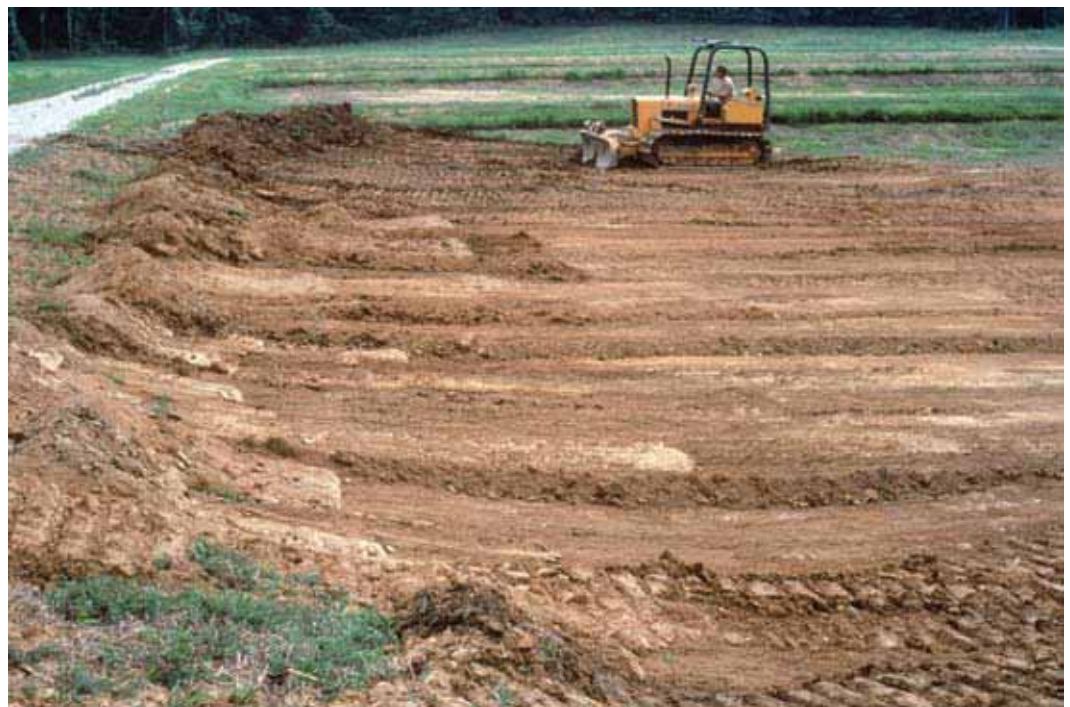
Figure 7.18. Sediments from the pond bottom itself should be the first source of soil for rebuilding levees and filling low areas.
