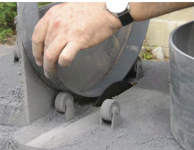
Figure 6. Cutting the ring to hold the mesh onto the silo.
