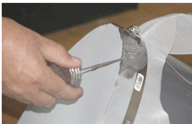
Figure 15. Apply PVC glue liberally.
