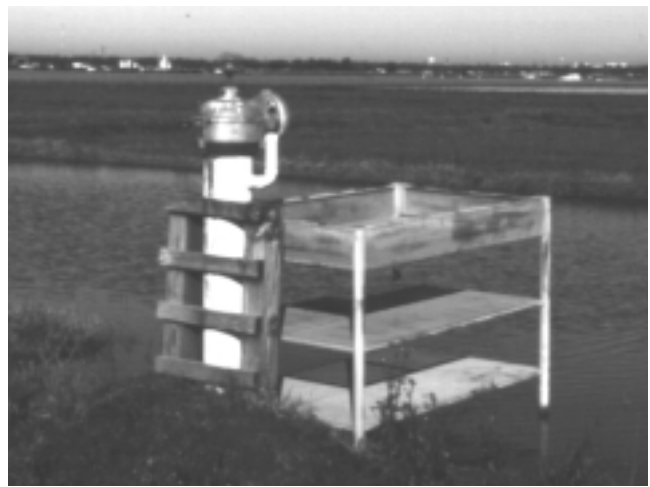
Well or relift circulation pump with screen aerator.
