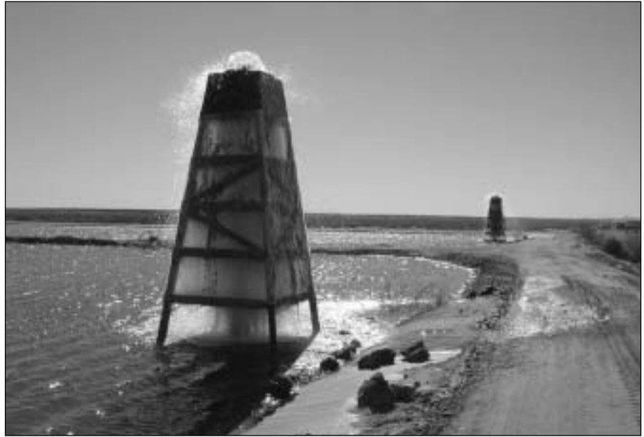
Figure 1. Degassing tower (courtesy of T. Samocho)
