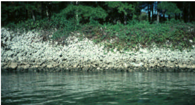
Stone rip-rap provides shoreline protection and fish habitat.
