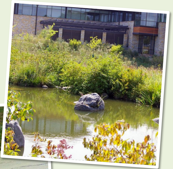
Rain gardens reduce runoff and prevent pollutants from reaching an urban pond.
