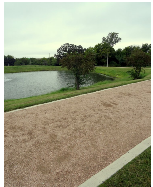
Use permeable surface, such as gravel or pebbles, to allow surface water to absorb into the ground rather than washing straight into the pond.
