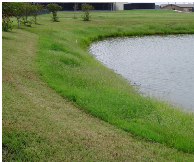
Creating a no-mow buffer zone as well as a gentle 3-1 slope around the pond's edge can significantly slow down surface flow before it reaches the pond, giving chemicals and sediment time to settle out.
