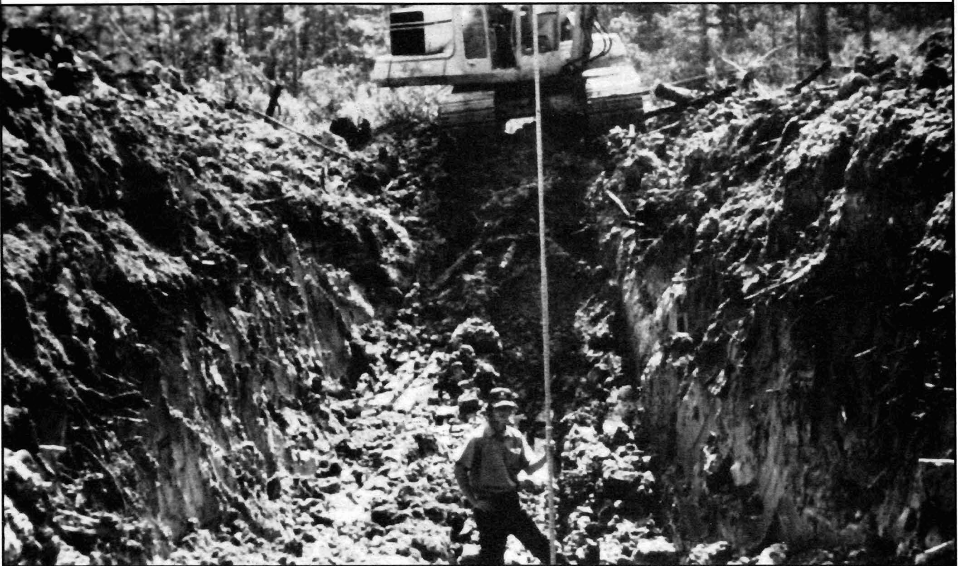
Cutting a trench for the clay core of the pond dam.
