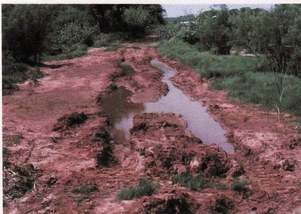
Roadway flooding often occurs near beaver ponds.
