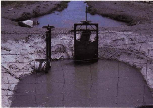
It may be necessary to install concrete aprons around headgates and tubes to prevent muskrats from burrowing next to them.
