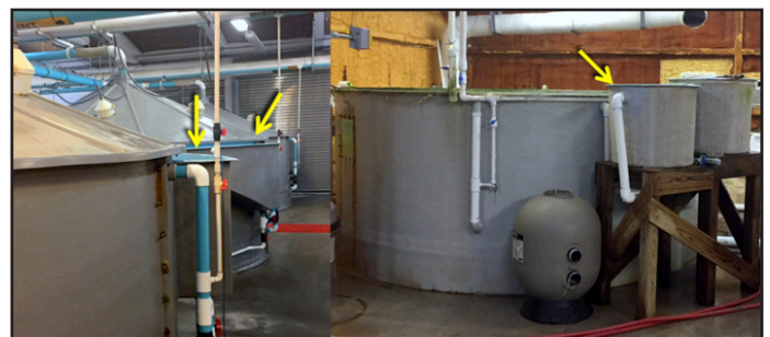
Figure 7. Egg collection at most hatcheries is accomplished by means of side mounted egg collectors positioned at water level on the side of the spawning tanks. A circular water flow in the tanks created by return water from the filtration systems pushes the buoyant eggs outward toward the sides of the tank and eventually through the opening of the egg collector. Different styles of side mount collectors can be seen in the image above at Texas Parks and Wildlife Department’s Sea Center Texas Hatchery in Lake Jackson, TX (left) and a commercial hatchery near Palacios, TX (right).
