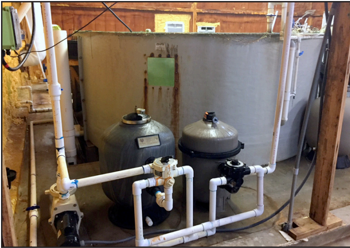
Figure 5. The “standard” spawning tank most commonly used at hatcheries measures 12 feet (3.7 m) in diameter and holds approximately 3,400 gallons (12,870 L) of water as seen in the image above at a commercial hatchery in Palacios, TX. A spawning system in commercial facilities is typically comprised of a pair of spawning tanks with a shared bioreactor tank filled with biomed, a 1.5 horsepower centrifugal water pump, one or more large bag or canister pre-filters, and an appropriately sized sand or bead filter.
